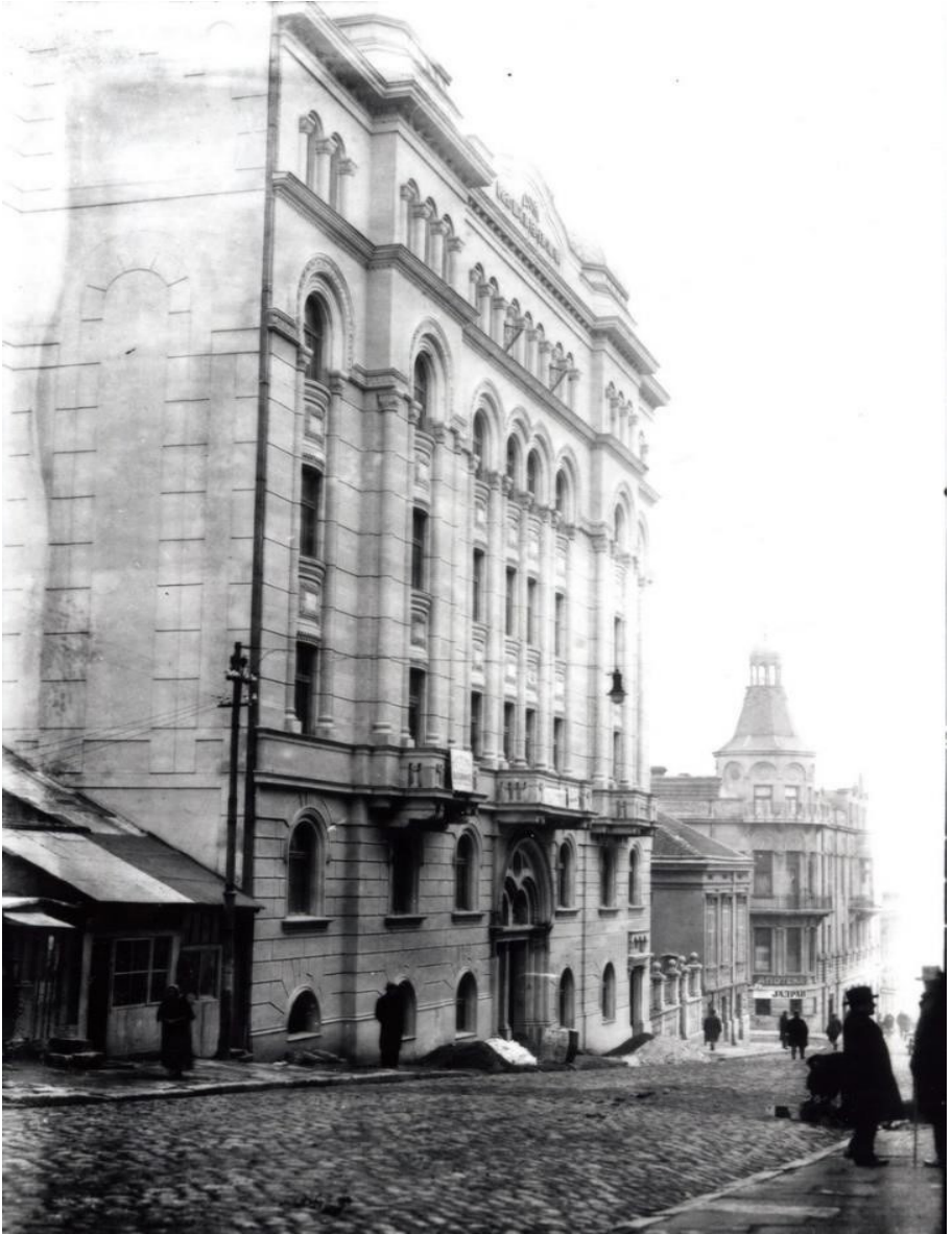
Figure 3. The House of the Jewish Church-School Community in Belgrade after its completion in the 1930s, showing the street's slope. (Photo from the Collection of Miloš Jurišić)
