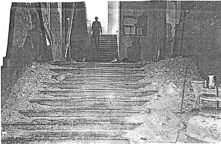
Sl.12. Oštećeno ulazno stubište u zgradu Židovske općine u Zagrebu, Palmotićeve 16, nakon eksplozije podmetnute bombe 19. kolovoza 1991. godine. Snimila Jasminka Domaš Damaged entry staircase to the building of the Jewish Community in Zagreb after the explosion of planted bomb on August 19, 1991 (photographed by Jasminka Domaš)
