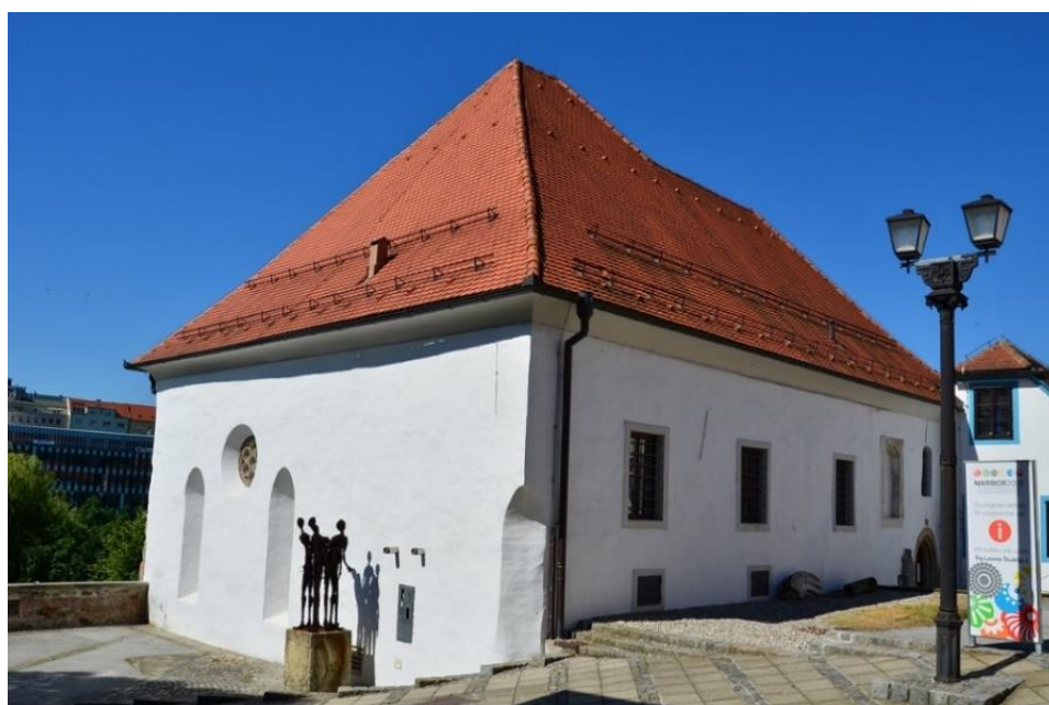
Figure 1. Maribor Synagogue, view from the northeast. Exterior. Photo: Janez Premk.
