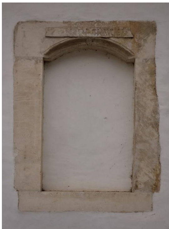
Figure 4. Built-in window on the northern façade with the dedicatory inscription of the Druckher couple, who purchased the building after the expulsion of the Jews in 1497 and turned it into All Saints Church. Photo: Janez Premk.
