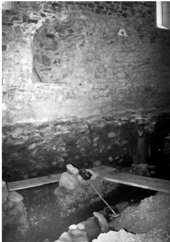
Figure 12. A niche in the southern wall of the hall. Interior. Photo: The Maribor Regional Office of the IPCHS, Fond Maribor—Sinagoga.
