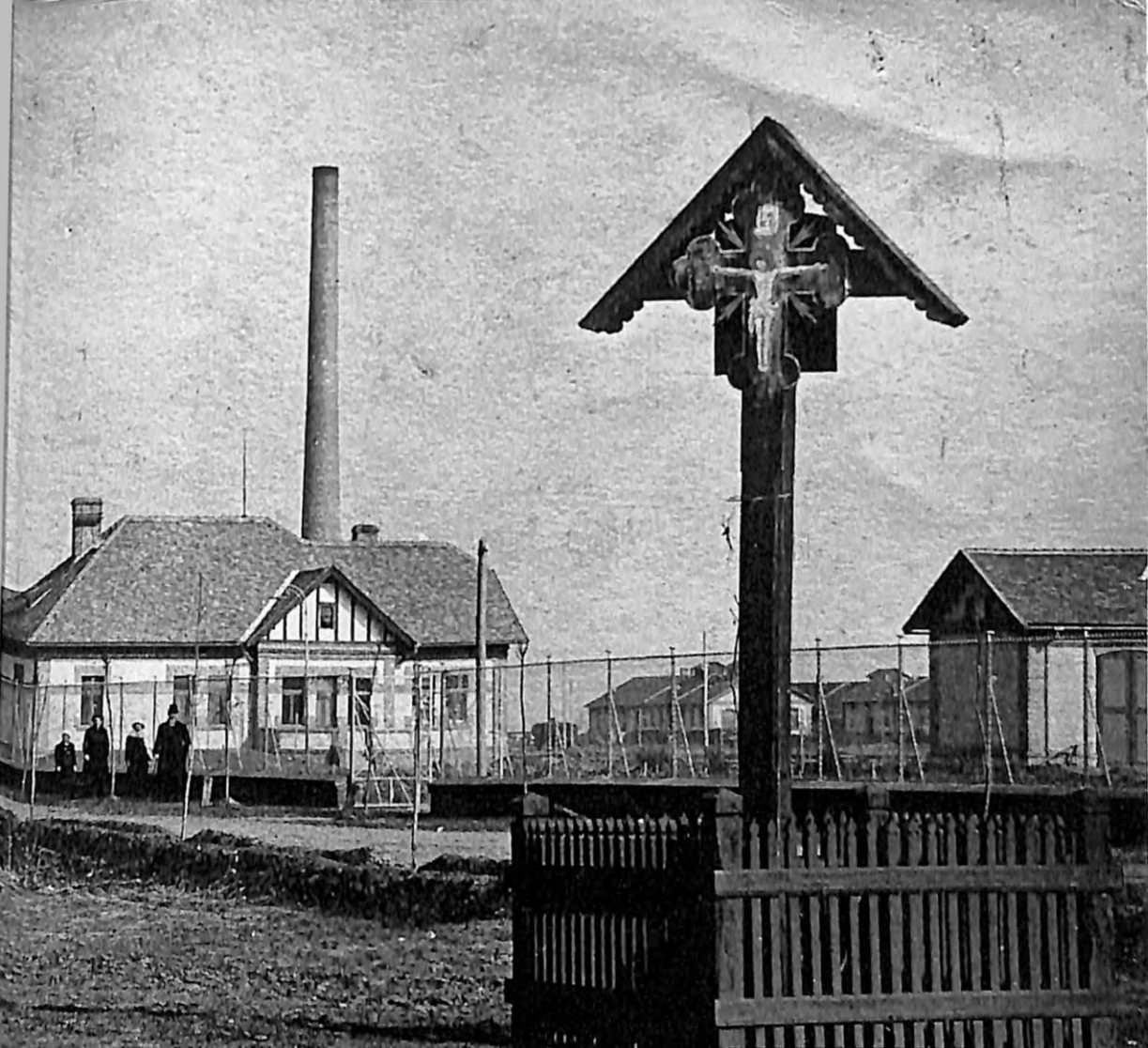
Kompleks šećerane, 1910-ih The Sugar factory complex, 1910s Ferenc Nemet
