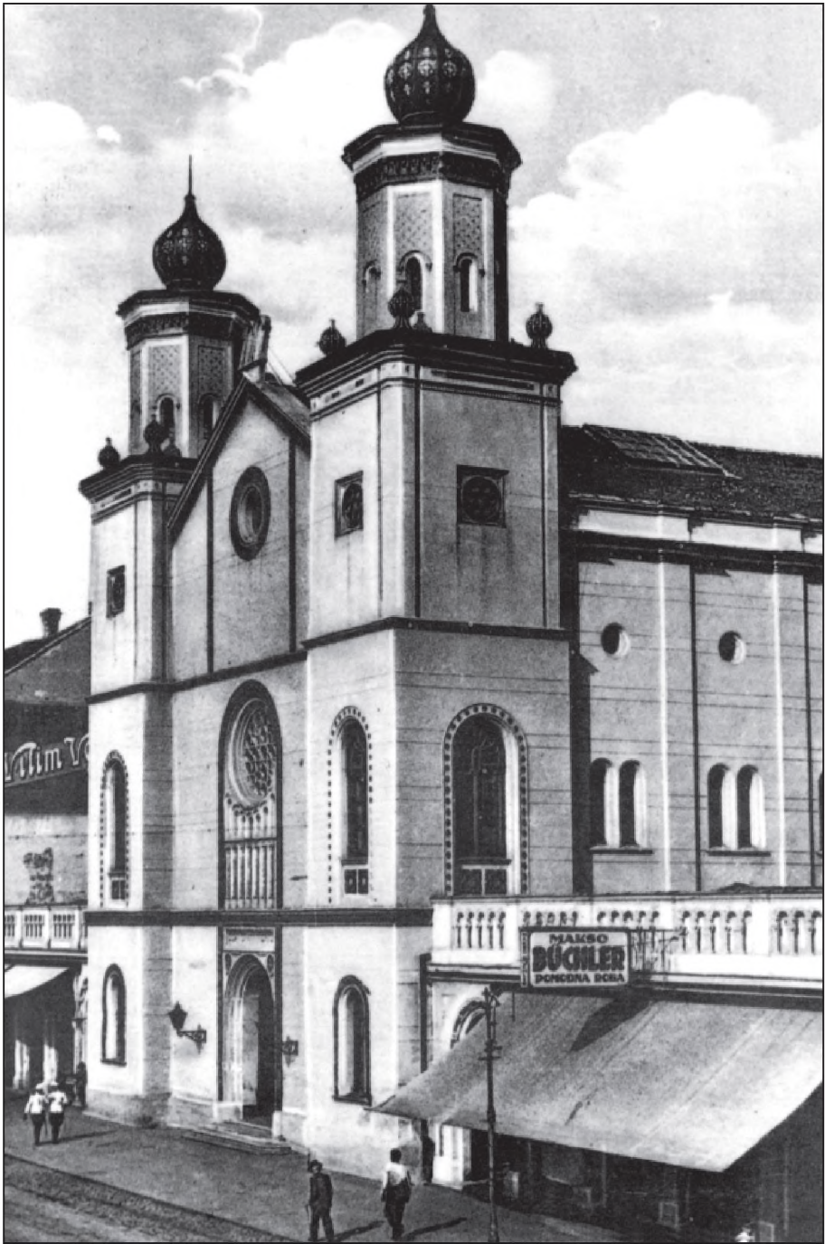
Synagogue in Osijek (1869), destroyed in World War Two
