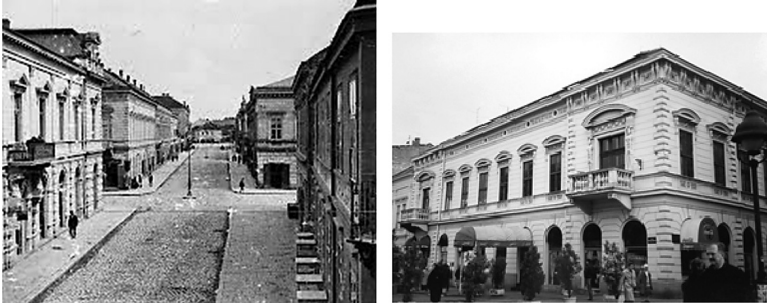
Figure 6. The old 19 th century buildings in Knez Mihailo street
