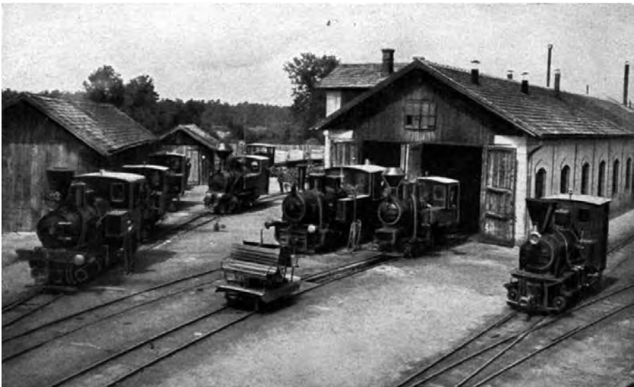
Boiler room of the company Našička d.d. in Đurdenovac and forest railway locomotives, Našice Homeland Museum
