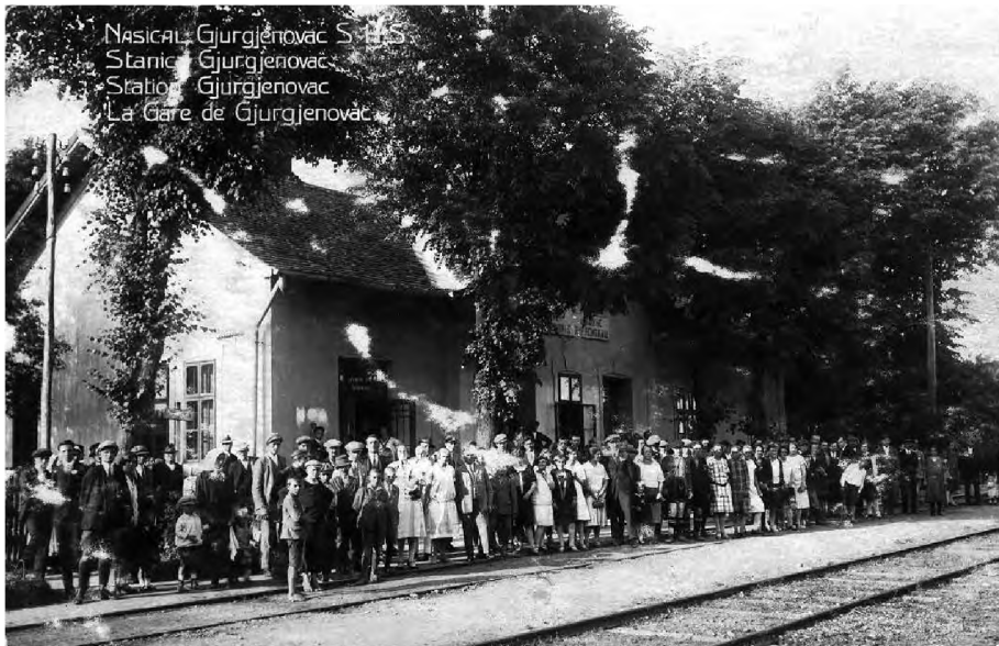
Railway station in Đurđenovac on the line Zagreb – Osijek, Našice Homeland Museum
